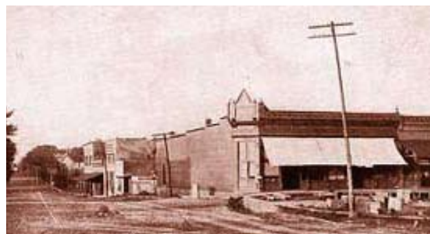
Intersection of Pine & McClurg – Richland, MO
